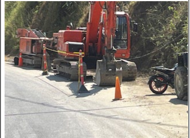
Photo 48: Improved housekeeping at work site, follow-up visit January 2024
