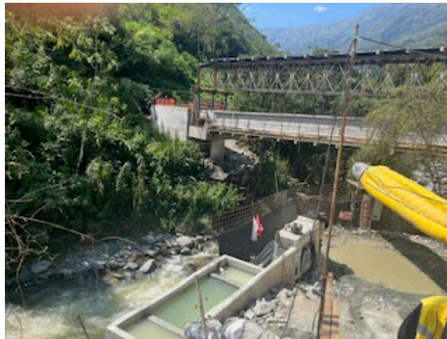
Photo 47: Improved retention of sediments at upper tunnel portal, follow-up visit January 2024
