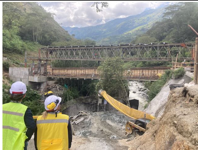
Photo 16: Bridge across San Andrés River and upper tunnel portal below
