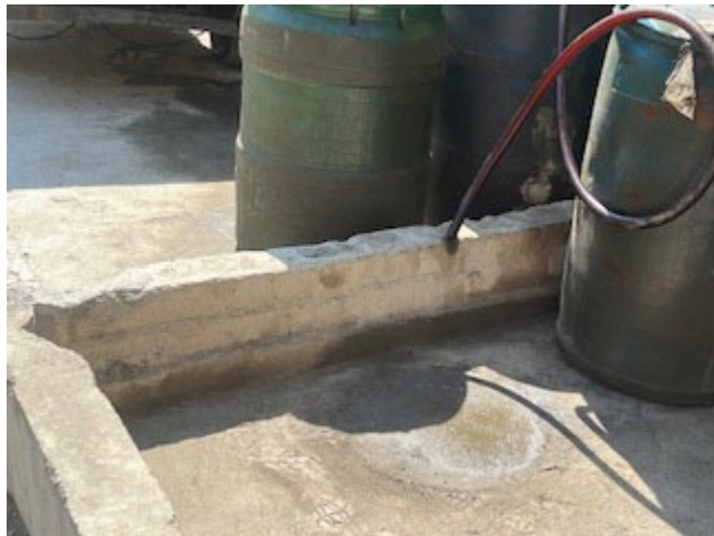
Photo 46: Improved oil containment, follow-up visit January 2024
