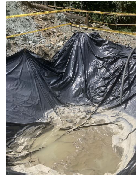
Photo 57: Temporary sediment trap at lower tunnel portal
