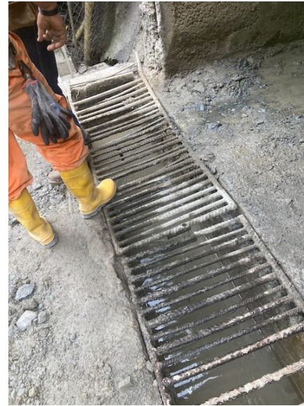
Photo 56: Drainage at lower tunnel portal
