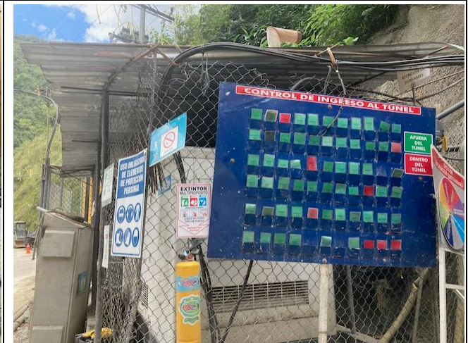
Photo 54: Control of workers' presence in tunnel
