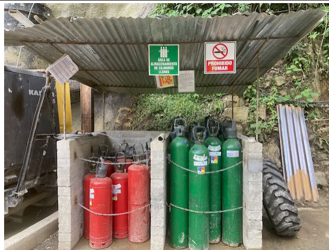
Photo 52: Gas bottle storage at tunnel portal
