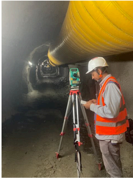
Photo 55: Control of alignment in tunnel construction
