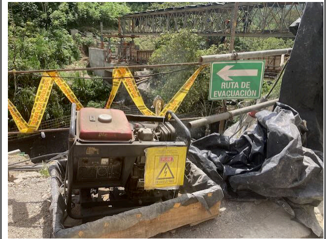
Photo 42: Construction equipment with inadequate containment 1
