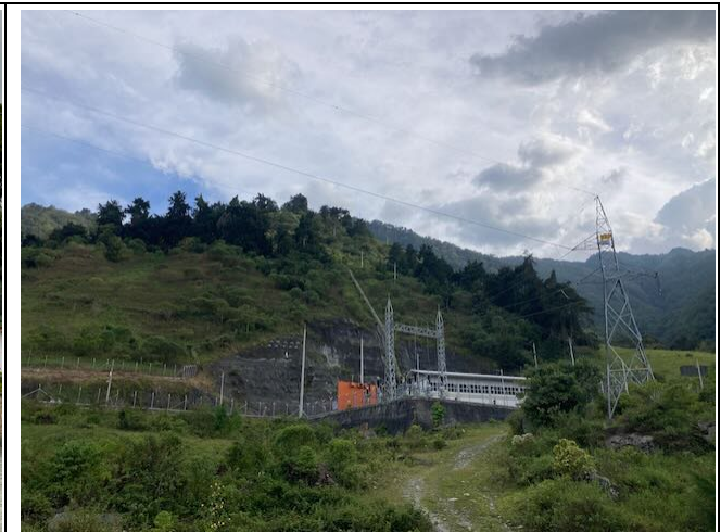
Photo 3: Powerhouse of Celsia's upstream San Andrés HPP
