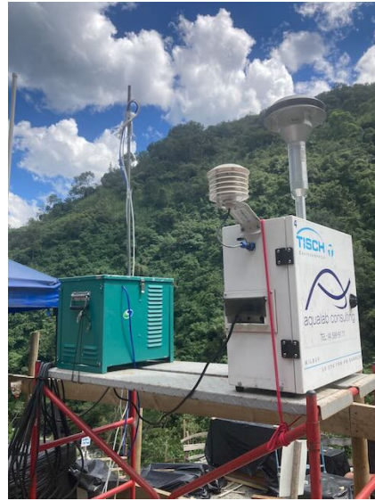
Photo 62: Monitoring equipment at powerhouse construction site
