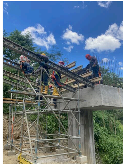
Photo 65: Workers with PPE for work at heights
