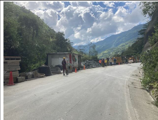
Photo 17: Space restricted worksite on highway near upper tunnel portal
