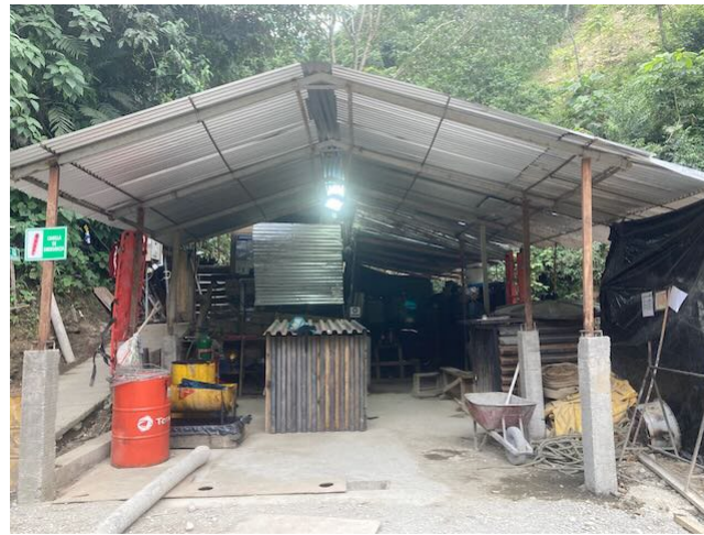
Photo 41: Equipment storage and worker rest area at lower tunnel portal
